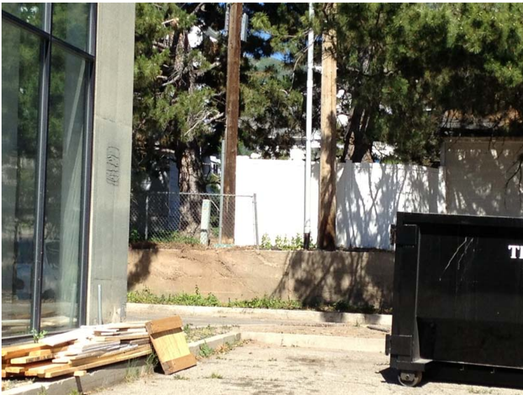
View of east property line (adjacent to residential). Chain link fence would be removed by a condition of approval.
